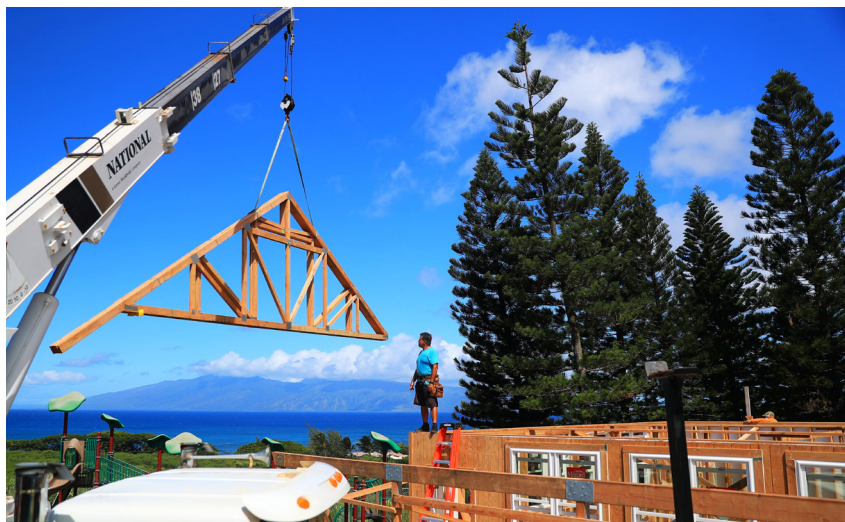
Left: A roof truss is lifted into place for the Graham Center for Creativity, Innovation, and Entrepreneurship
